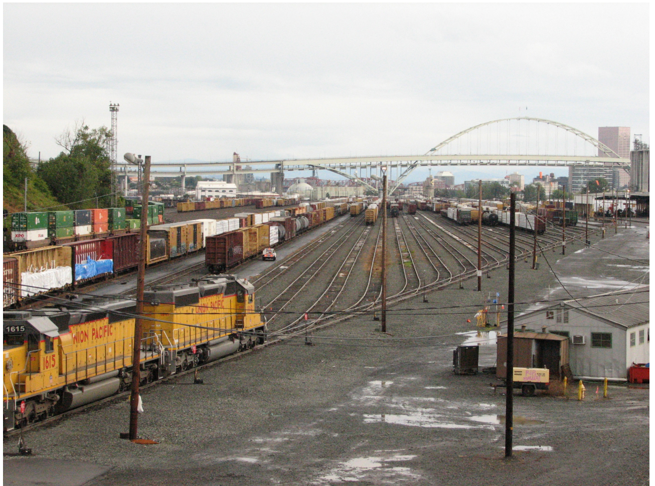
Union Pacific's Albina Yard looking south taken in 2019. (Photo by "Graywalls" | CC-SA4.0I.)
