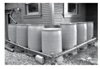
There are several common pitfalls to avoid when installing a rain barrel system. Starting out right and taking your time with installation and fittings will pay off in the long run. Since rain barrels are typically installed in-line with an existing downspout, it lives right next to the foundation of your home. Any clogs or leaky connections can cause stormwater to drain into a basement window well or into a crawl space, certainly areas
