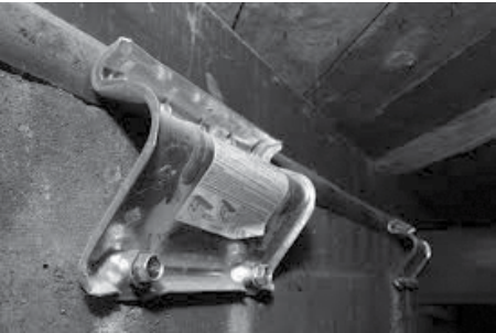
Bracket used to bolt a home to it's foundation
