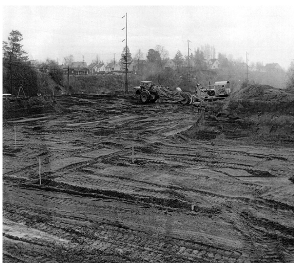
Preparing the foundation for Kaiser Hospital by tamping down the earth circa —1957.
